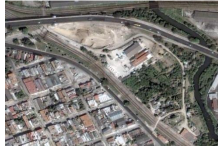
Figure 7. Construction of Upper Luyano Wastewater Treatment Plant with aerial image from Google Earth dated 2008 (top panel “a”) and design drawings from UNDP (2006b) (bottom panel “b”)
