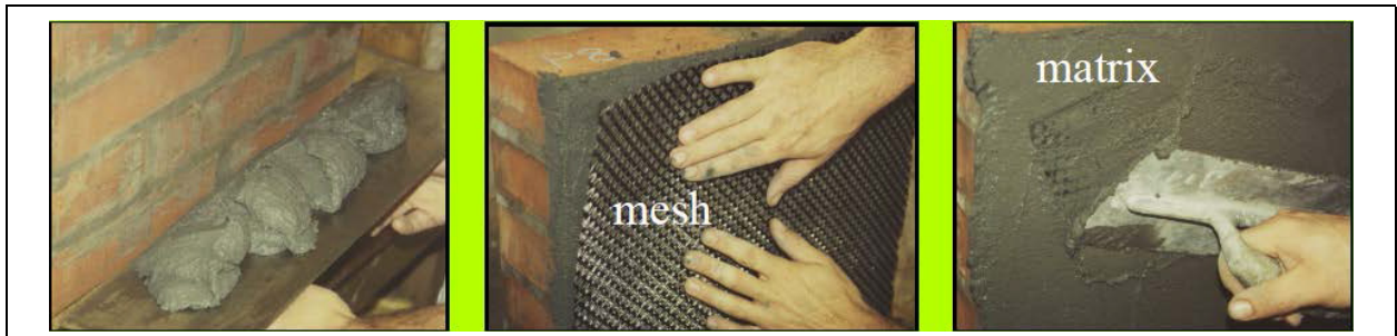
Figure 4. Application of FRCM on a masonry wall
