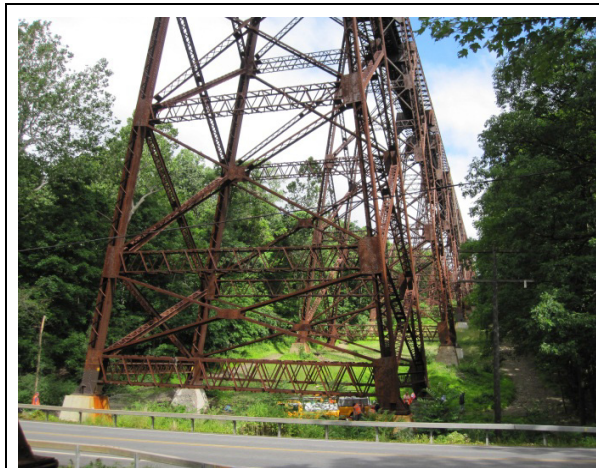
Figure 7. Structural steel trestle supported by trapezoidal concrete pedestals
