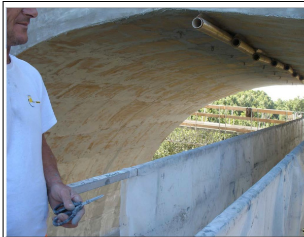
Figure 6. Rolls of fabric hang while scaffolding is advanced.
