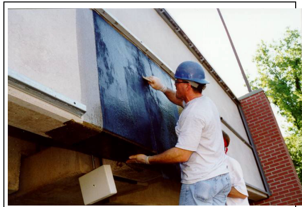
Figure 2. Examples of strengthening of historical and modern masonry with FRP
