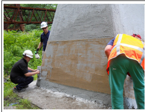
Figure 8. Application of PBO fabric over the cementitious matrix
