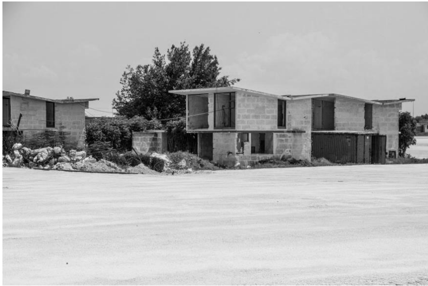
Figure 2. Yacht Club Residential Condominium, Varadero, Cuba
