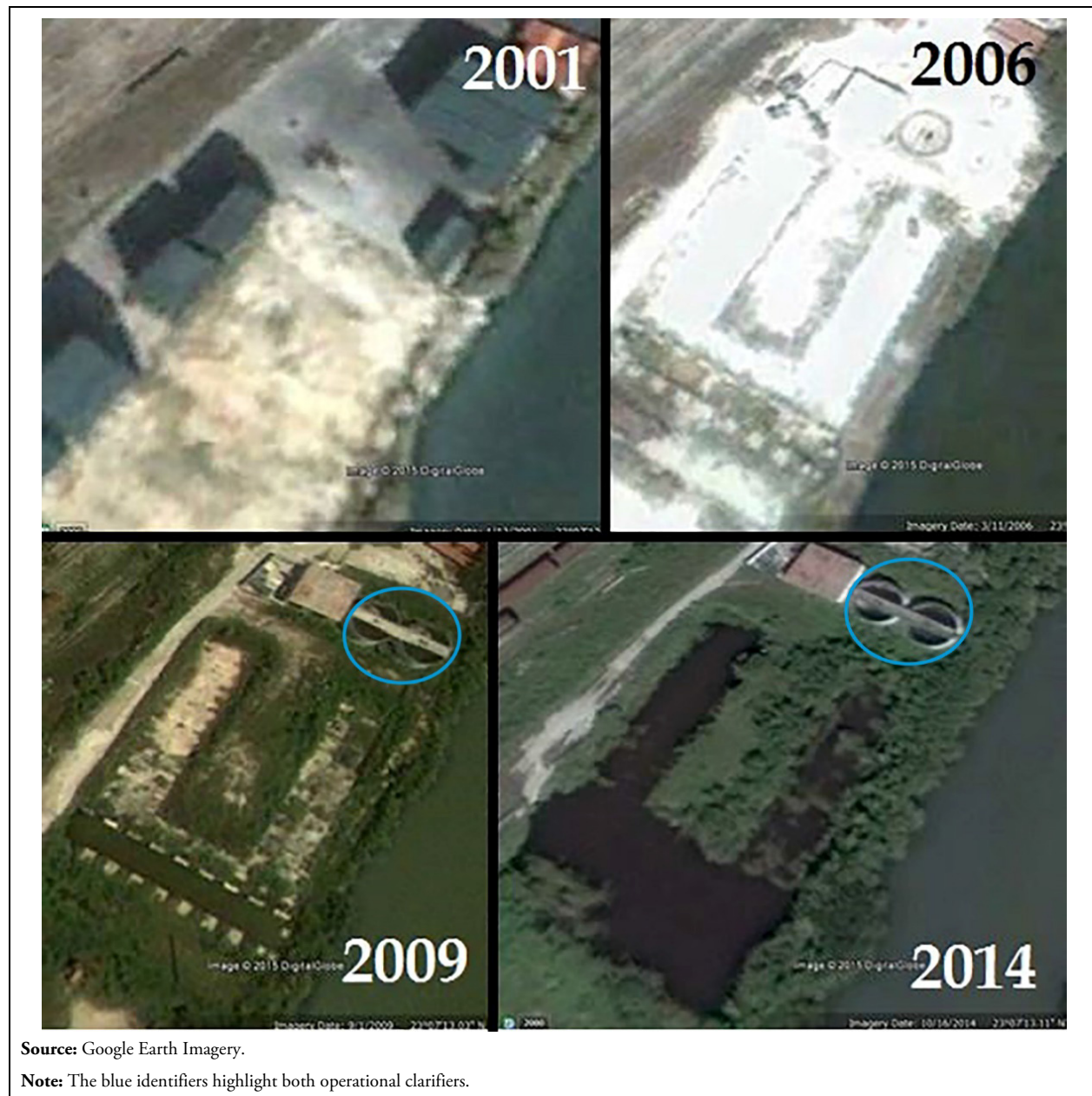
Figure 5. Lower Luyanó WWTP
